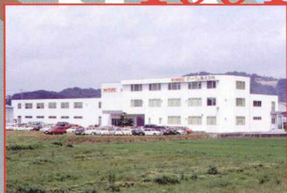
1991年3月 開発棟増設完成 March 1991 Expansion of development building completed.
