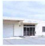
掛川支店 掛川市杉谷南2-1-10 Kakegawa branch office 2-1-10 Sugiyaminami, Kakegawa city
