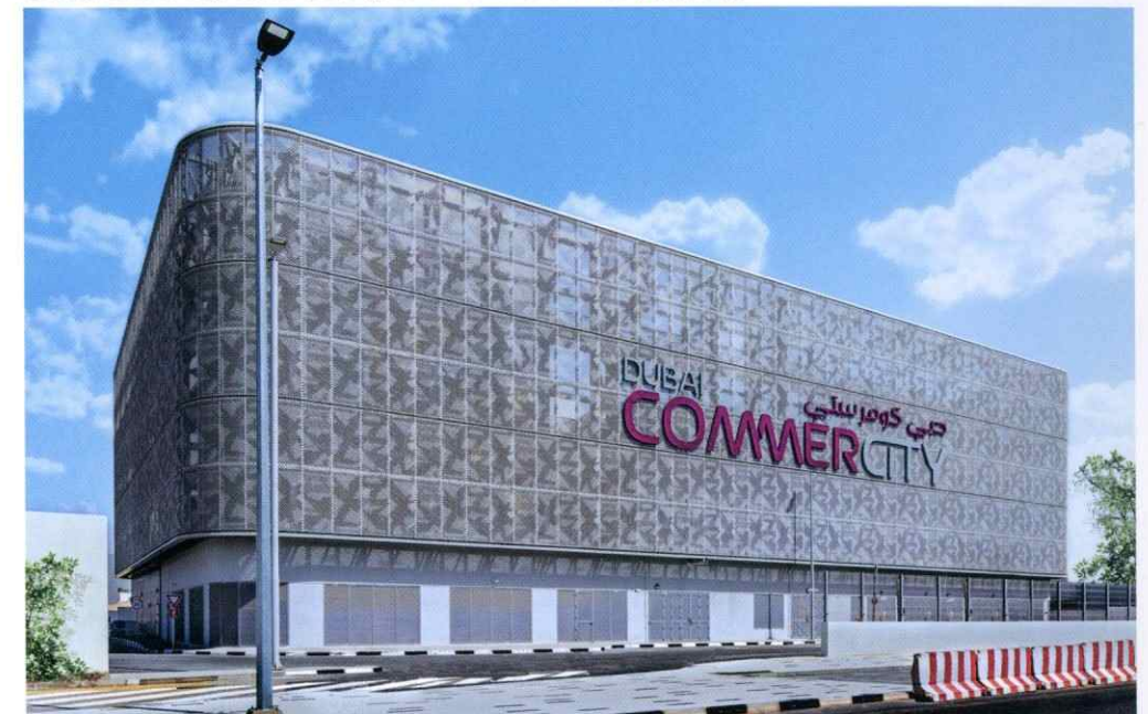
⑤ Dubai Commer City Central Utility Centre ■電気■情報通信■空調■衛生■内装
