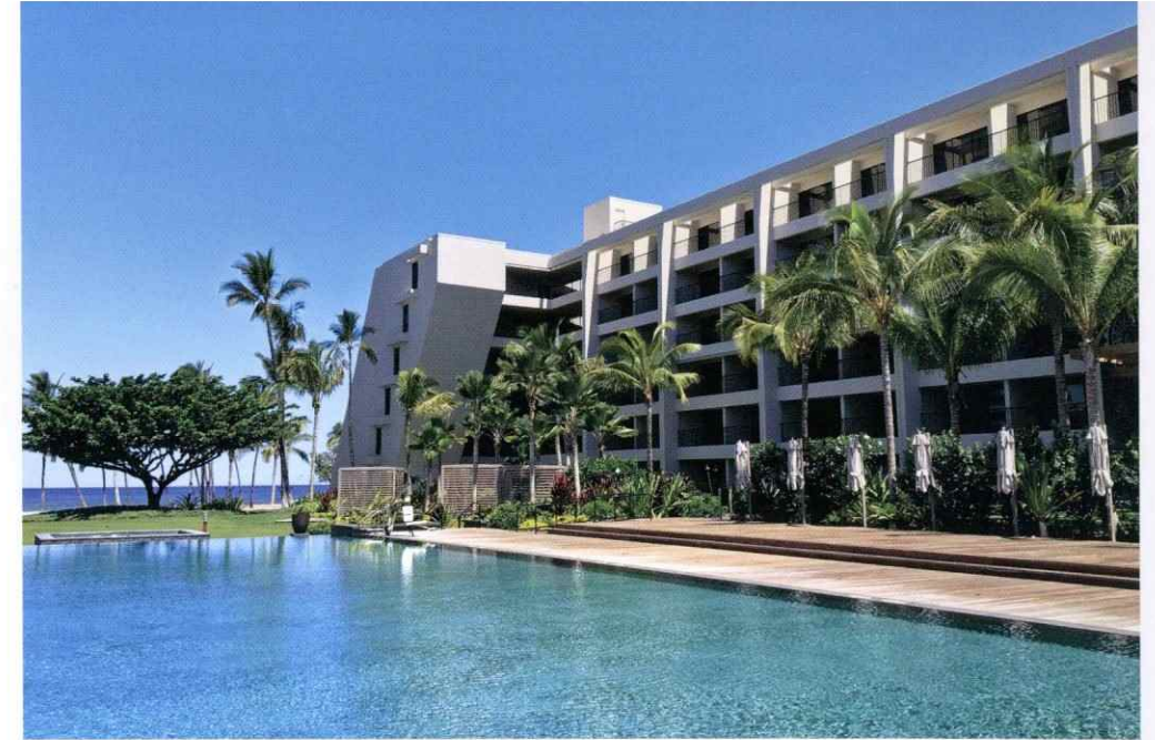
④ Mauna Lani Bay Hotel & Bungalows Renovation ■電気■情報通信
