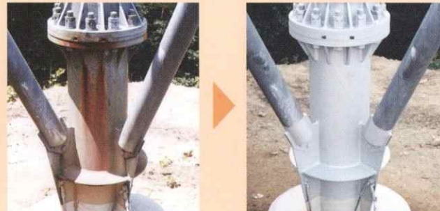
▲延命化対策例 Typical life sustaining measures
