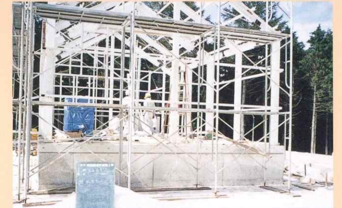
▲無線機器室組立工事 Construction of radio equipment rooms
