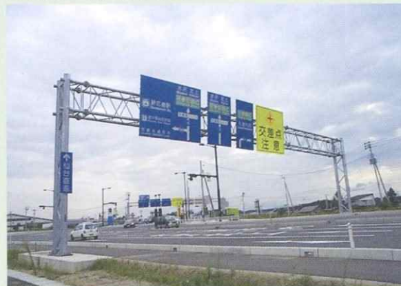
▼道路標識柱 Road sign structures
