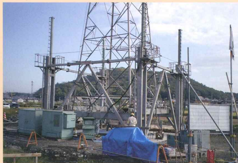
▲鉄塔かさ上げ装置 Tower lifting apparatus
