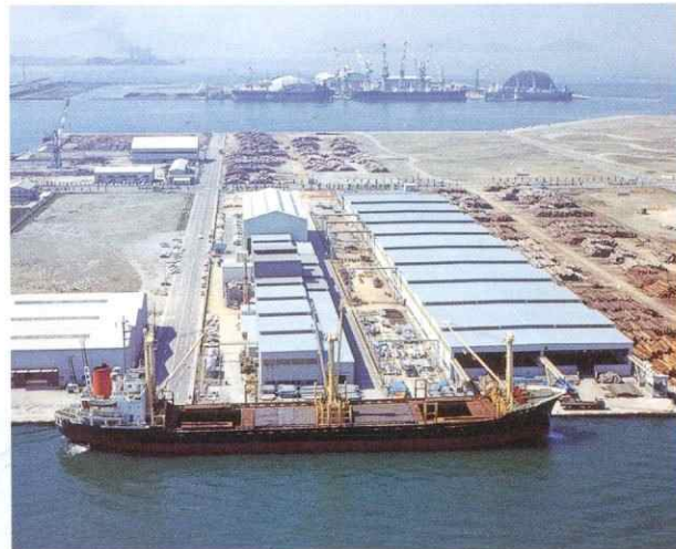
■丸亀東工場 (50,109㎡) Marugame East Factory
