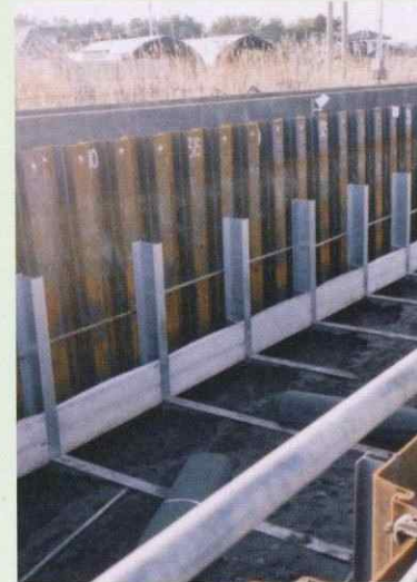
▲用水路 Irrigation canals
