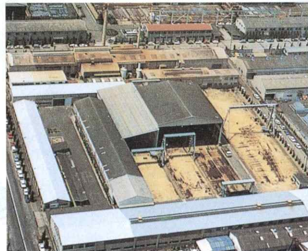
■丸亀西工場 (14,876㎡) Marugame West Factory
