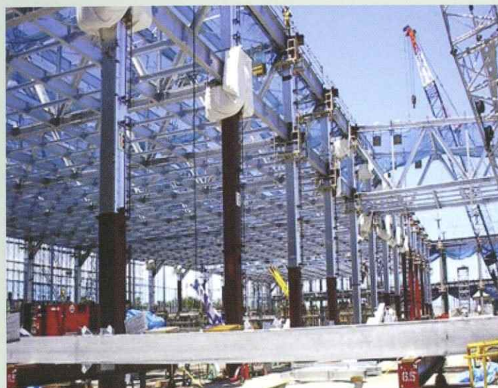
▲建築鉄骨 Building frames
