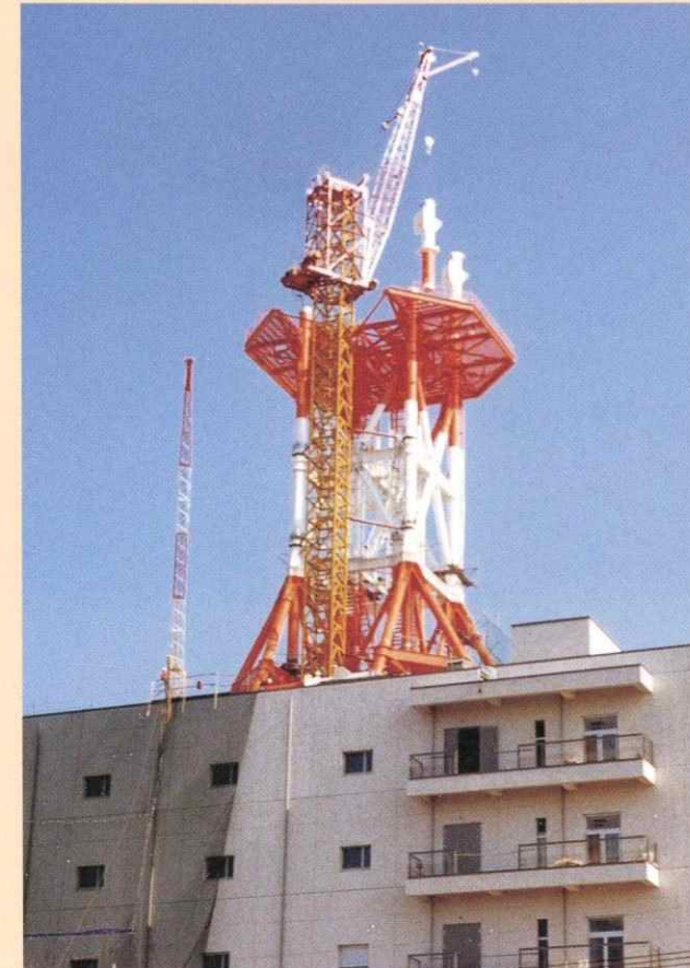
▲鉄塔建方工事 Construction of steel towers
