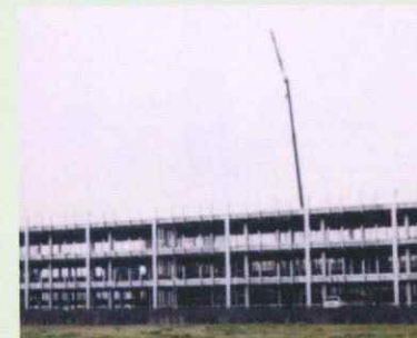
▲駐車場 Parking structures
