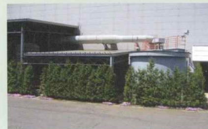
▲環境調和型廃水処理設備 Environmentally harmonizing waste water treatment facilities
